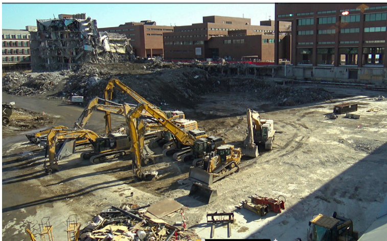
The demolition of the old Science Center is nearing completion.
