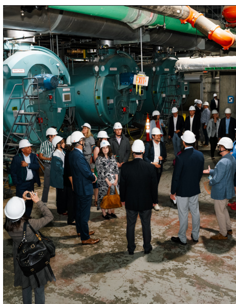
The Green Ribbon Commission took a tour of UMass Boston's pumped-seawater cooling system.
